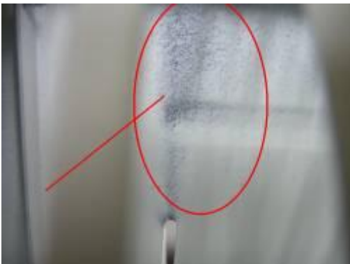
Photo-27 Poor painting of inner bracket buckle position.-2
