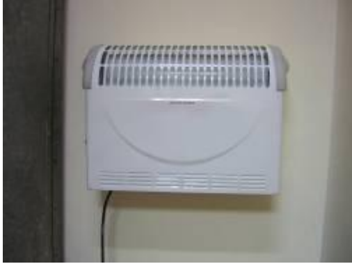
Photo-33 Use 6mm drill to make hole in the wall and drive in the concrete anchor, and then use the wood screw to fix the bracket and put the main unit on the bracket.
